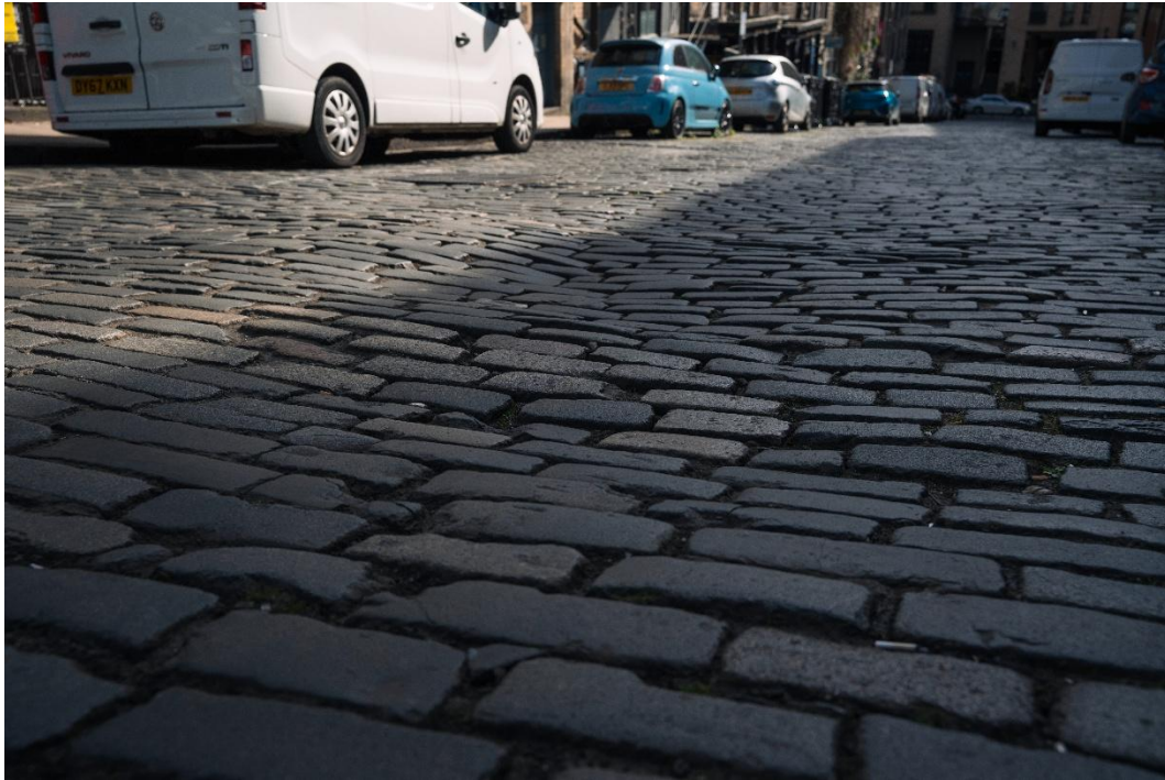
(Uneven cobbled surface on Blair Street)
